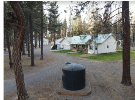
A well prepared home that survived the 14,000 acre "242" Labor day fire unattended. Photos courtesy of Chiloquin Oregon Fire & Rescue
